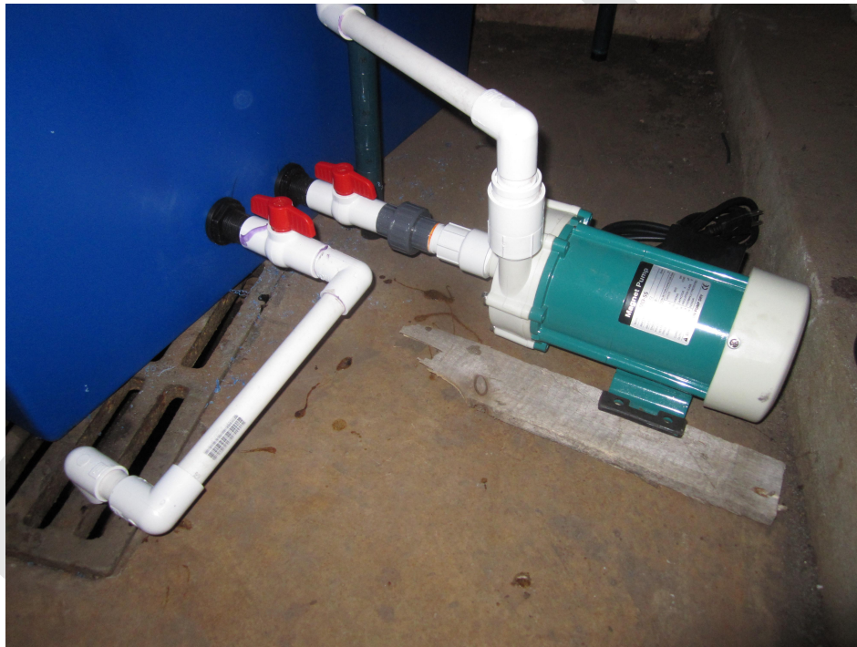
Figure 4. The bottom corner of the sump filter where the Iwaki® brand pump draws water from the filter and pumps it back to the top shelves of aquariums. A second bulkhead accommodates a quick drainage system for water changes. The bulkhead can be opened and the filter water drains into a storm drain below. For ease of replacement, note that there are union valves between the pump and the filter box. If the pump burns out, the unit can be removed via the union and replaced quickly and easily. Photo by Danté D. Fenolio.
